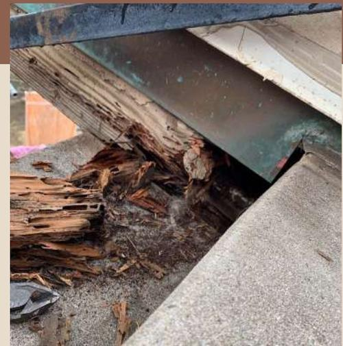
The sidings were torn open from two different areas and completely removed. The crevices were then cleaned, sidings replaced with treated wood and coated with a clear sealant to form a protective layer on the wood and concrete.
