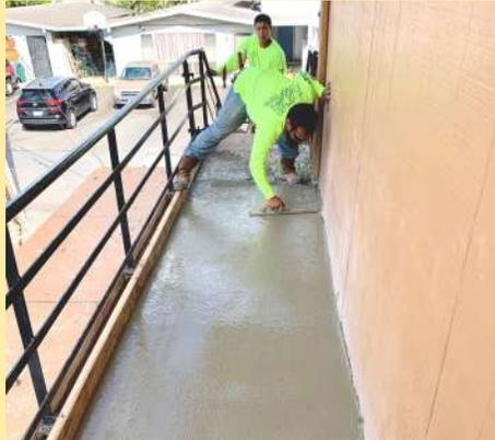
The second floor walkway is exposed to the elements, so a penetrating waterproofing sealant was applied to the concrete surface.
