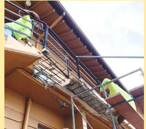
The existing reinforced steel rebars were removed due to severe rusting.
