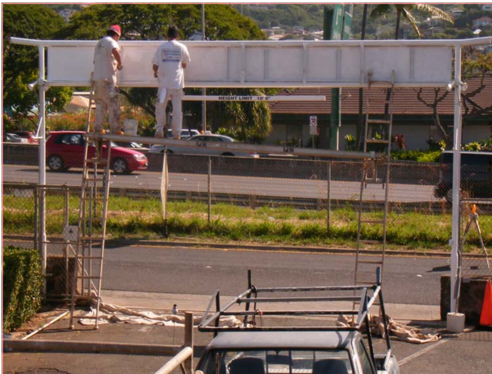
Scott Nakaoka and employee applying primer to the torii gate
